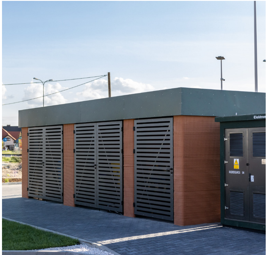
Pic. Photo of Poland's first building printed at a construction site in Wyszaków. The print was realized in close proximity to a transformer station.
